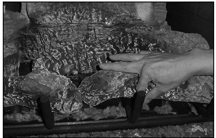
Figure 14.3 Placement of Rock Wool
