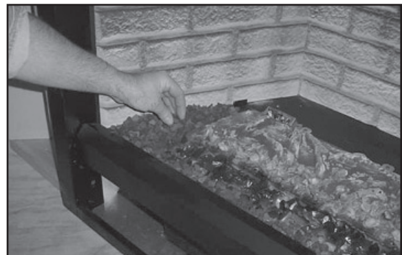
Figure 10.3 Placing the Lava Rock
