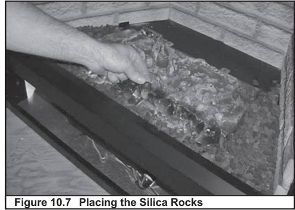
Figure 10.7 Placing the Silica Rocks
