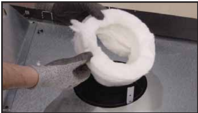
Figure 9.6 Remove the insulation from the outer vent pipe. For rear venting there is no insulation in the outer vent pipe.
