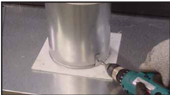
Figure 9.7 To attach the first section of vent pipe, make sure to use the fiberglass gasket in the manual bag to seal between the first vent component and the outer fireplace wrap. Use 2 self tapping screws to secure the gasket to the outer wrap.
