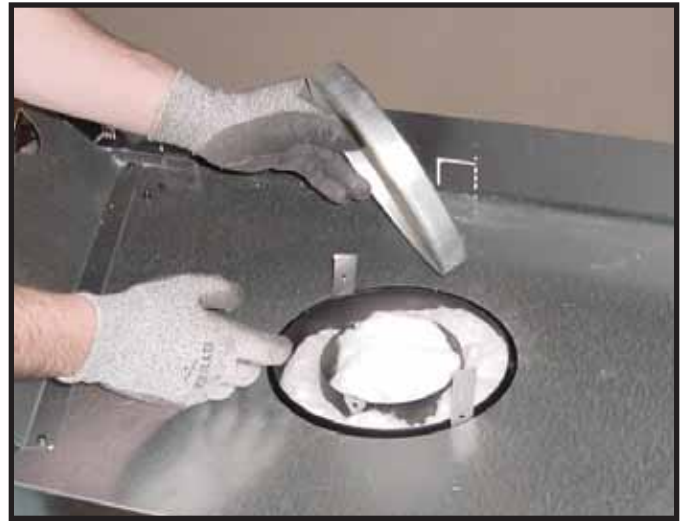
Figure 9.4 Remove the seal cap.
