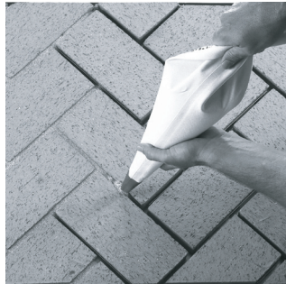
Figure 29 - Grouting Brick
