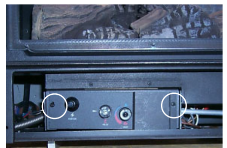
Remove the 2 screws holding the Control Panel in place.
