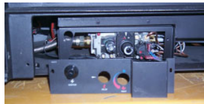
Remove the 2 screws holding the Control Panel in place.
