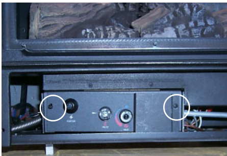
Remove the 2 screws holding the Control Panel in place.
