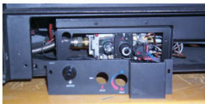
Remove the 2 screws holding the Control Panel in place.
