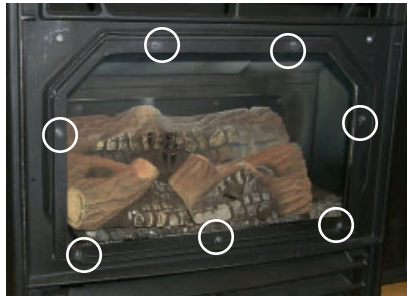
Remove the 7 nuts holding the Front Glass Bracket to the front face.
