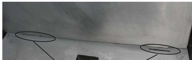
Slots on floor of firebox base.
