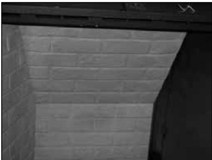
Figure 14.4 Install Upper Back Refractory
