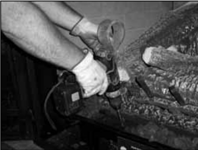
Figure 14.18 Installing Andirons
