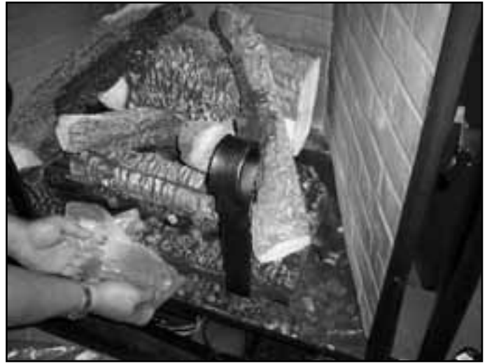
Figure 14.19 Placing Lava Rock
