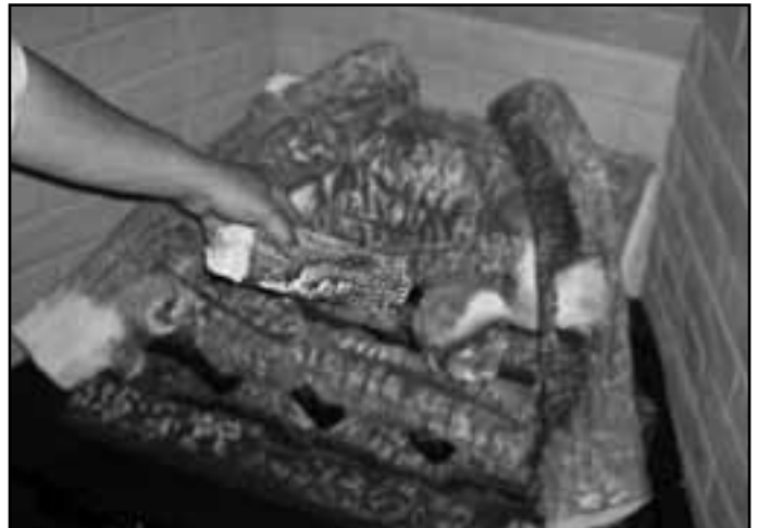
Figure 14.16 Positioning Left Middle Log
