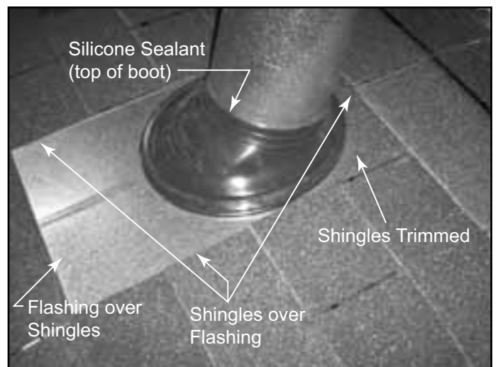
Figure 10.18 Installation Complete
