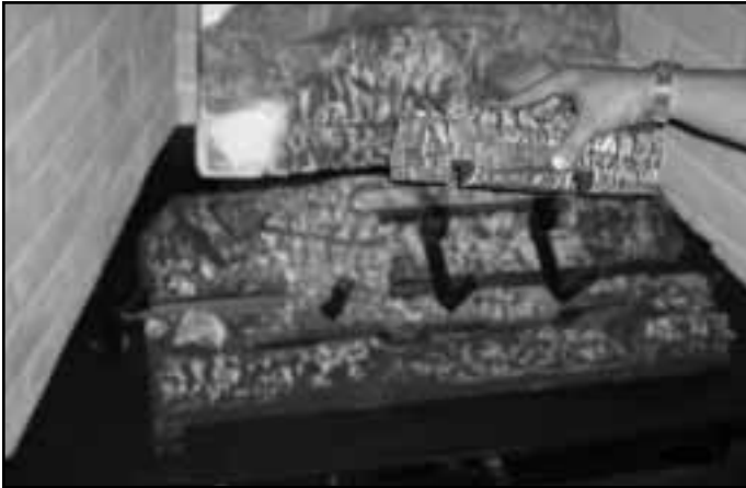
Figure 14.12 Positioning Right Front Log
