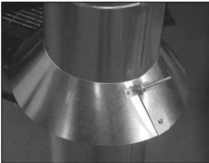
Figure 10.14 Assembling the Storm Collar Around the Pipe
