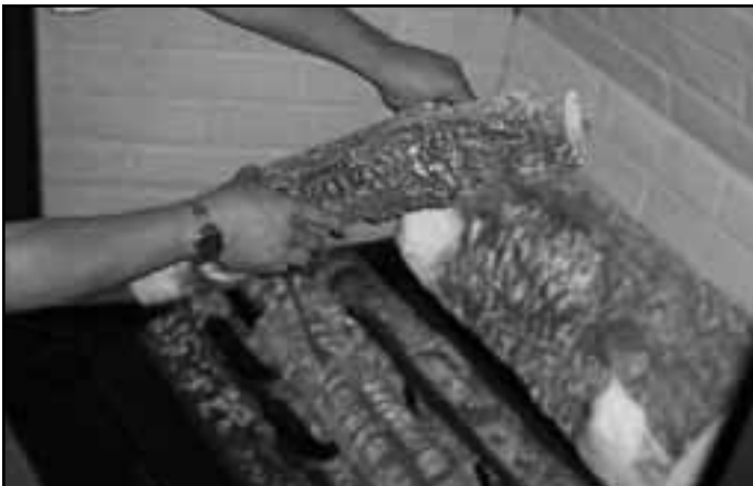
Figure 14.13 Positioning Left Log
