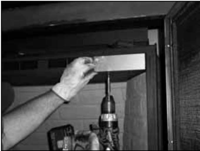
Figure 14.7 Adjust the Vertical Baffle
