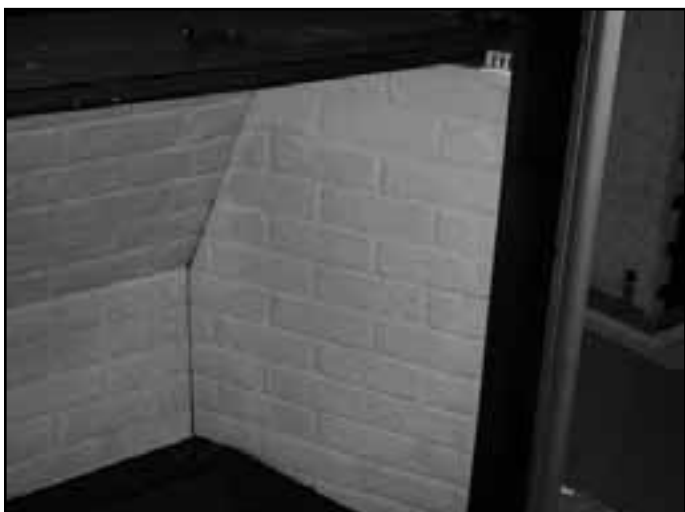
Figure 14.5 Install Right Side Refractory
