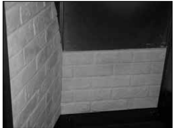
Figure 14.3 Install Lower Back Refractory
