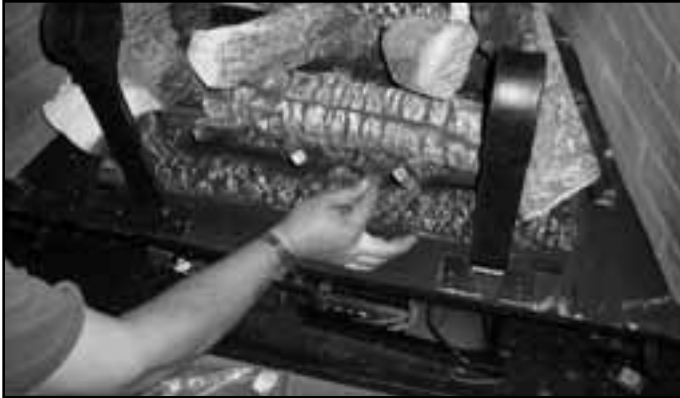
Figure 14.17 Placing Rockwool
