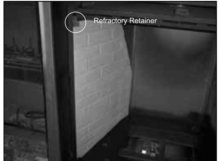
Figure 14.2 Install Left Side Refractory
