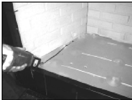
Figure 12.2. Using a saws-all, cut out the floor.
